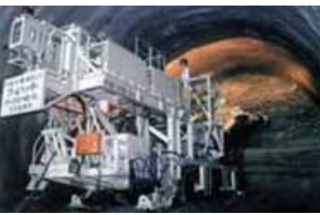
Kindaich Tunnel of JR East, 2001
