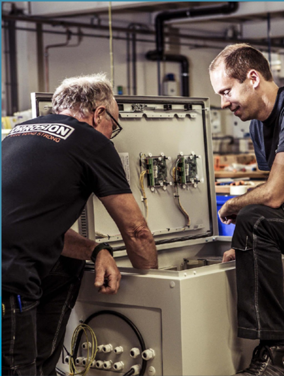
Assembly of a power cabinet. Image courtesy of CORROSION. All rights reserved.
